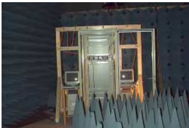
Figure 8: Sample data system, front view (UTP equivalent)
